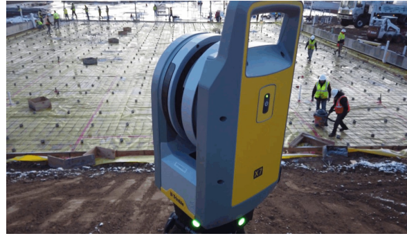
3D laser imaging scan during concrete placement
